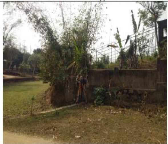
4. Total Station at embankment & plot corner
