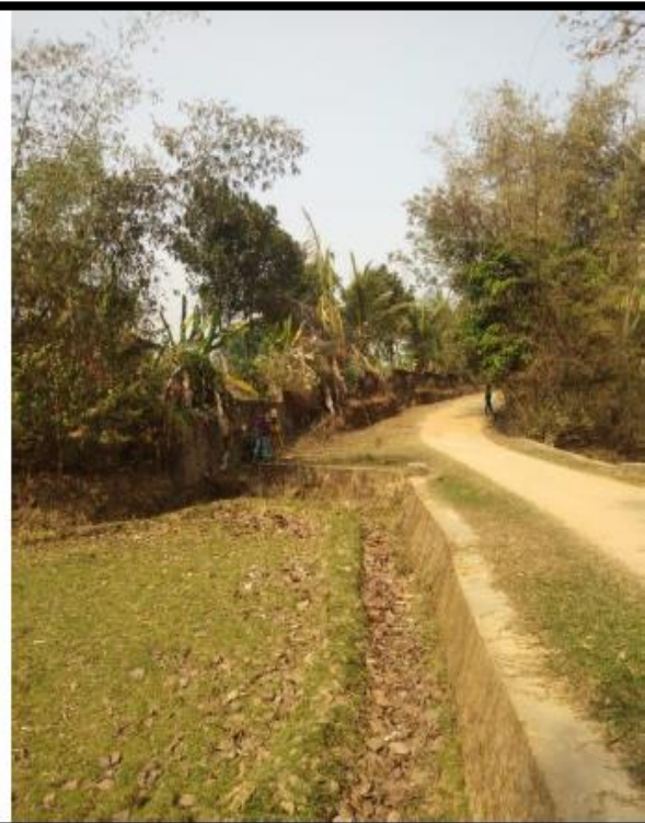
2. Protection embankment west of approach road
