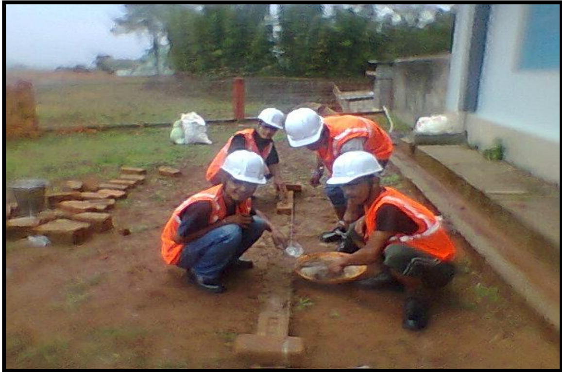
Fig: - Masonry Student
